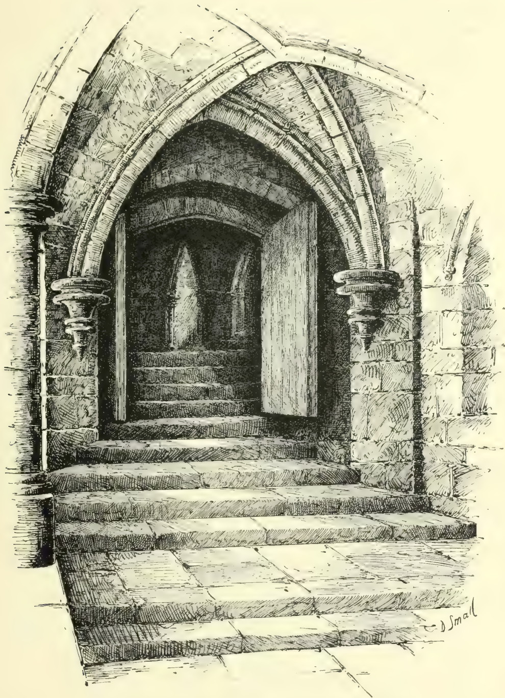
Stair from South Aisle of Lower Church, leading up to Nave.
